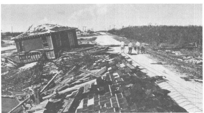
Though this house remained intact, the force of a coastal flood knocked it off its foundation, causing extensive damage. conceivably can be included in building codes in regard to flooding. For example:
